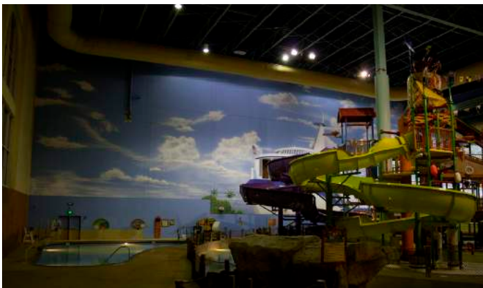
BEFORE — 400W Highbays
