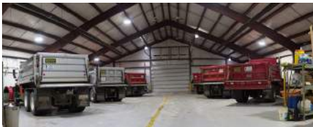
AFTER: PHX22-145 Installed
