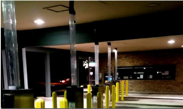
BEFORE — 250W Metal Halides
