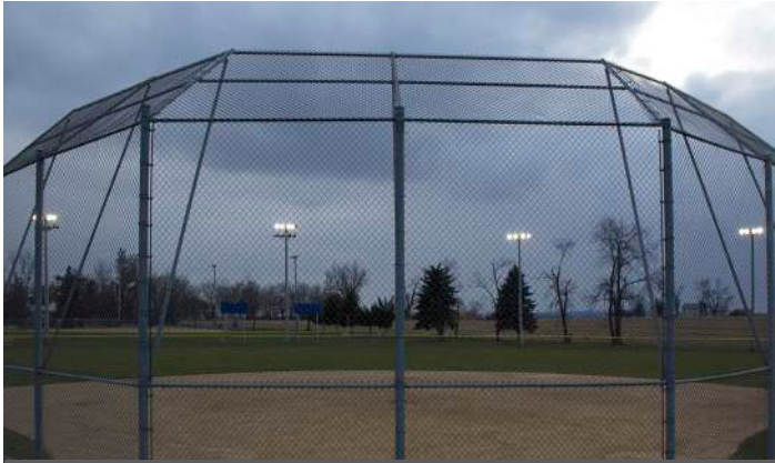
BEFORE - 1000W Metal Halides
