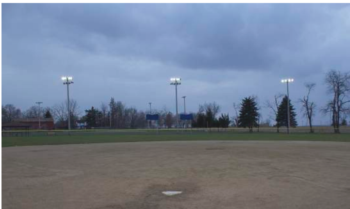
BEFORE - 1000W Metal Halides
