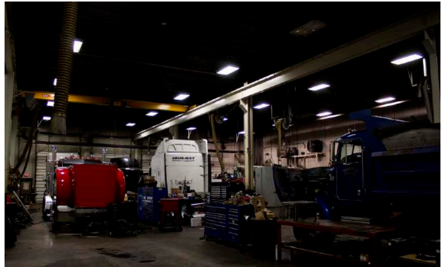
230W PHX LED HIGHBAYS INSTALLED (5,000K Version)
